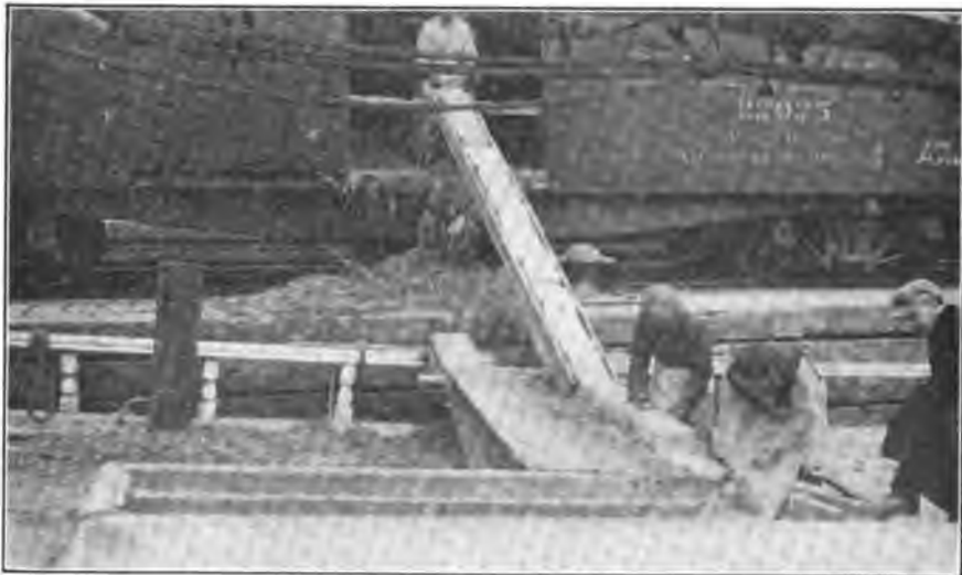
FIG. 149.—Loading firebrick shipped in bulk from cars to schooner. Fourteen cars carrying 200,000 brick, weighing 700 tons, in shipment.
